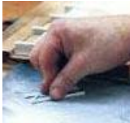
Figure 9: Floor, Step 3: sanding knife cuts
