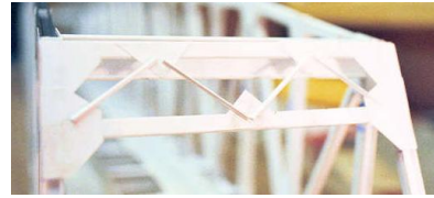
Figure 28: Portal bracing
